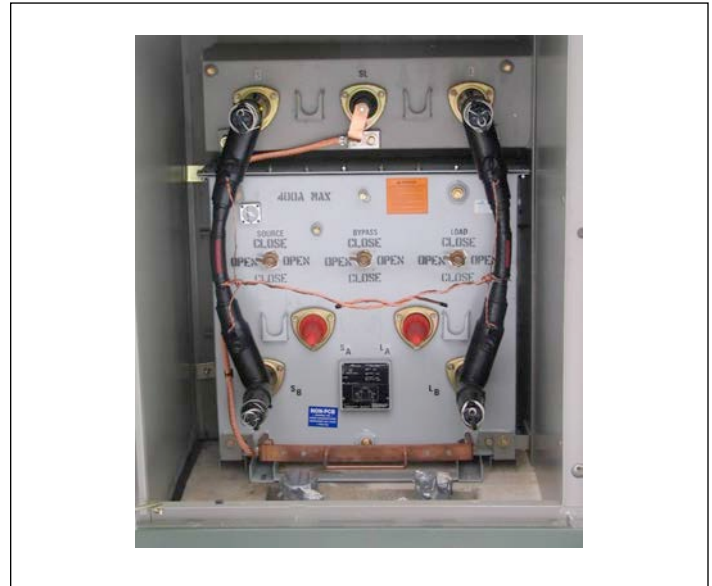
Figure 7. Voltage regulator bypassing operation
